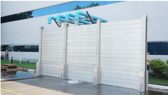
Watertight Wall Assembly Training
