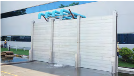
Watertight Wall Assembly Training
