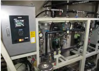
Membrane Filtration Facilities
