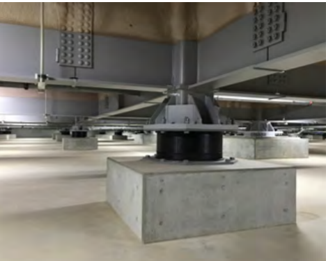
Adoption of Seismic Isolation Structure Including Ancillary Areas (ROHM Apollo Chikugo Plant)
