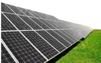
Solar power generation systems
